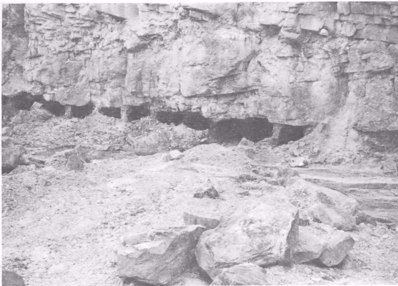
TYPICAL AUGER OPENINGS SECTION G, STRIP AREA R FIGURE 35
