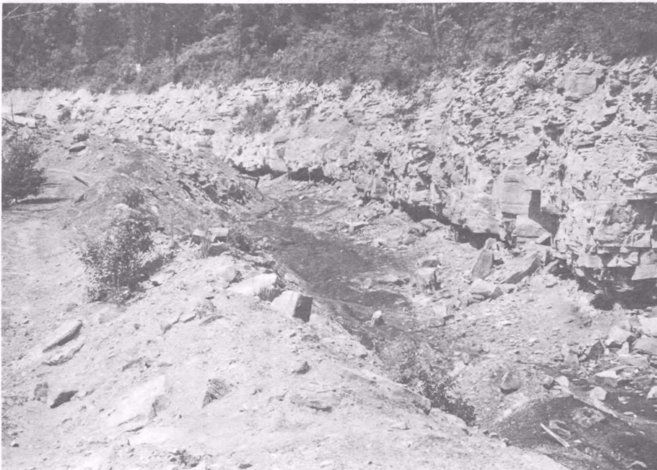
FRACTURED HIGHWALL RESULTING FROM EXTENSIVE AUGERING SECTION G, STRIP AREA R FIGURE 36
