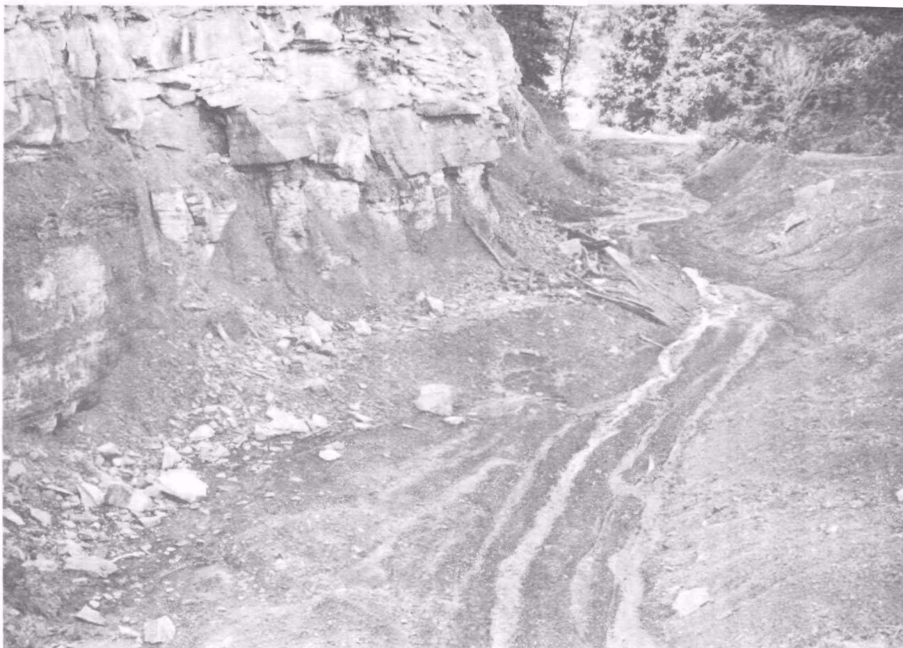
HIGHWALL AND BENCH SHOWING SURFACE WATER RUNOFF SECTION C, STRIP AREA C FIGURE 23
