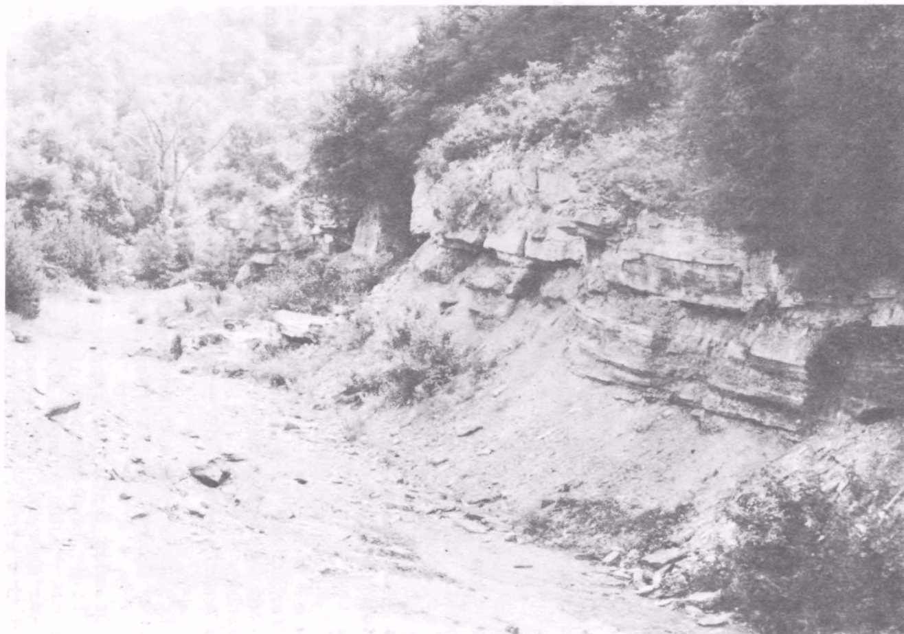
TYPICAL REVERSE TERRACE BACKFILL SECTION F, STRIP AREA B FIGURE 27
